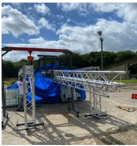
Figure 22: Ramp deployment at Vernon
